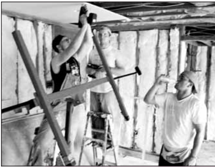
Concordia University Nebraska students rebuild housing.
